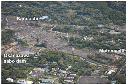
Photo1 Kandachi area after disaster (photo taken on Oct 16, 2013 by PASCO CO. & SECOM CO. LTD)
