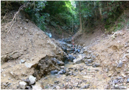
Photo 3 Nanjo No.3 area photo (Bed erosion)
