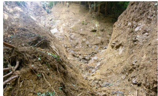
Photo 2 Nanjo No.2 area photo (Bed erosion)
