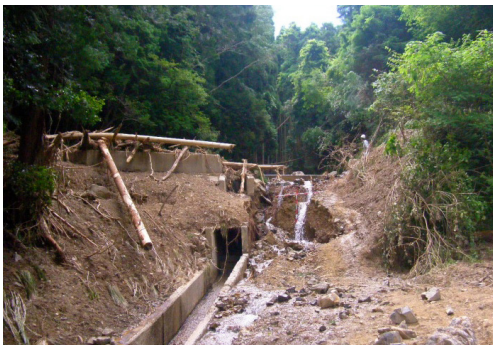
Photo 5 Nanjo No.5 area photo (Reservoir construction)
