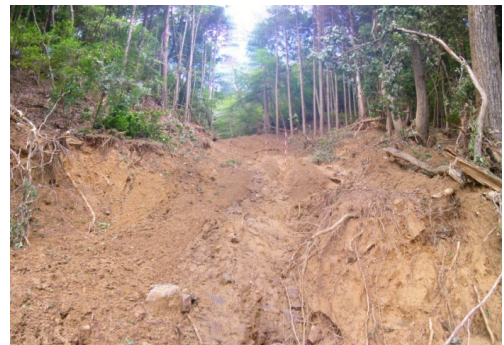
Photo 1 Nanjo No.1 area photo (Landslide)
