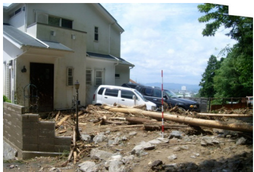
Photo 7 Nanjo No.7 area photo (Damaged house)
