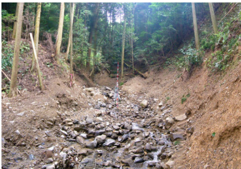
Photo 4 Nanjo No.4 area photo (Bed erosion)
