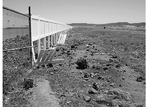
Photo 24 A damaged fence enclosing runway in Tafuna Airport.
