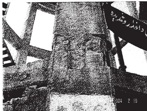
Photo 12 Concrete column and rebar on the east side of the water tank shown in Photo 11
