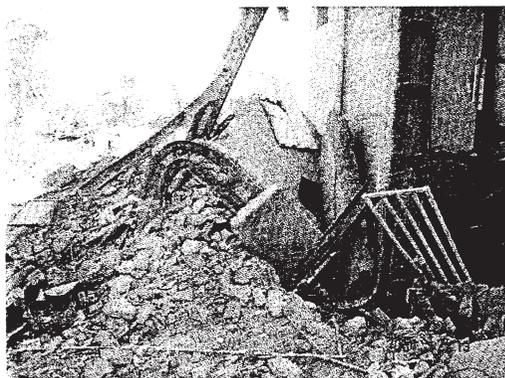
Photo 13 Collapsed steel frame building near by the water tank. This building was dislocated about 1.3 meters westward (rightward)
