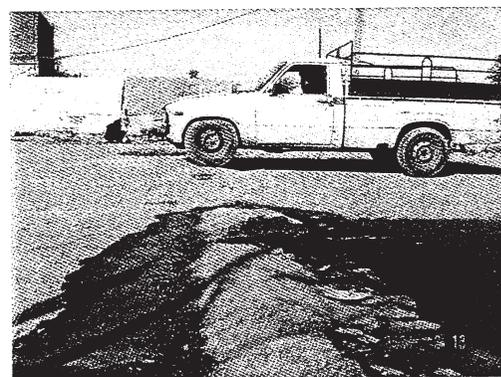
Photo 14 Bulge on a traffic road due to water hose underneath
