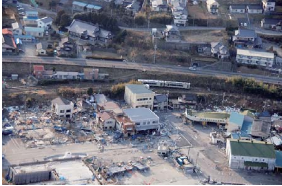
Photo 2. Ofunato-Line • Ofunato-Shimofunato (Provided by JR East)
