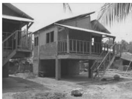
Fig. 12 Fishermen's safer house in Pangandaran Village constructed by MMAF (Photo from MMAF, 2006)
