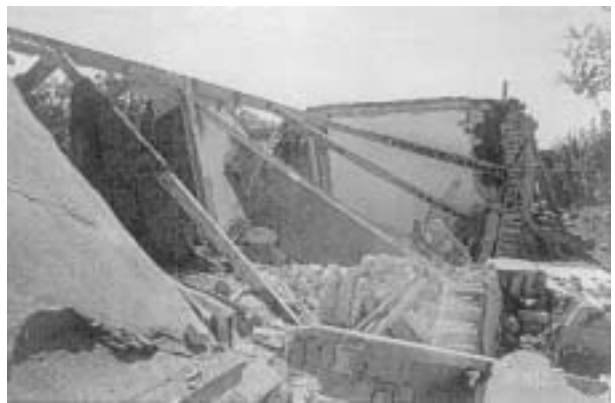
Photo 3 A typical collapsed URM building with a Jack-arch floor slab (Changureh)
