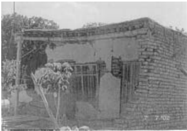
Photo 2 A thatched timber roof bonded with asphalt (Tablashkin)
