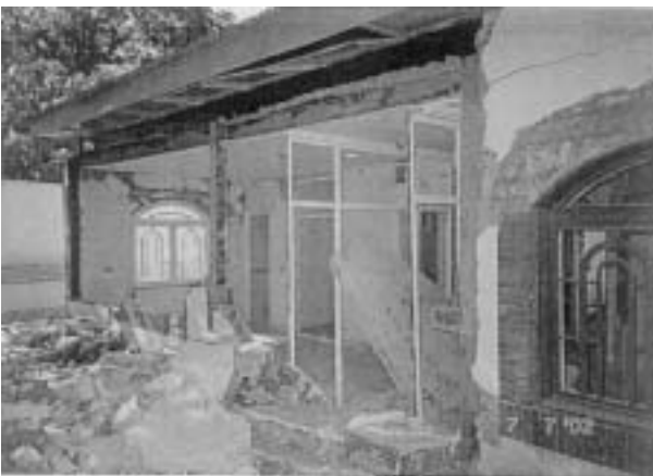
Photo 6 Out-of-plane failure of the infill of a semi-steel structure house (Changureh)
