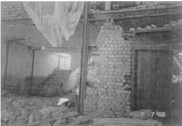
Photo 5 A surviving semi-steel structure with a Jack-arch floor slab (Changureh)
