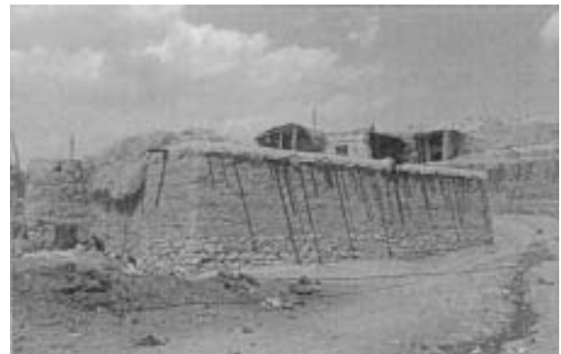
Photo 9 View of the adobe test house
