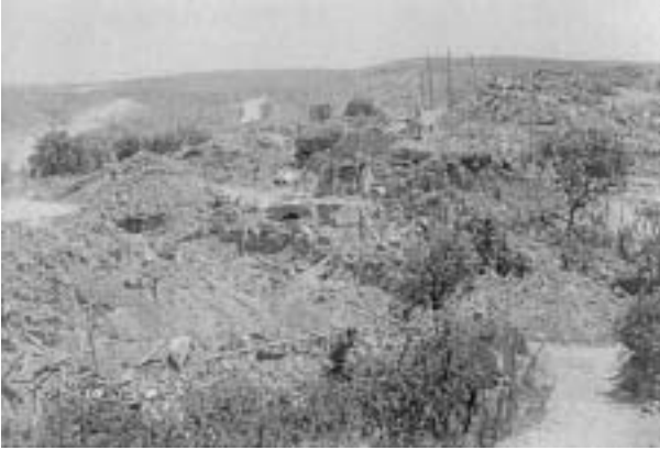
Photo 1 Collapsed adobe buildings which had arched and/or timber roofs (Abdareh)
