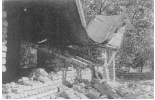
Photo 3 A typical collapsed URM building with a Jack-arch floor slab (Changureh)
