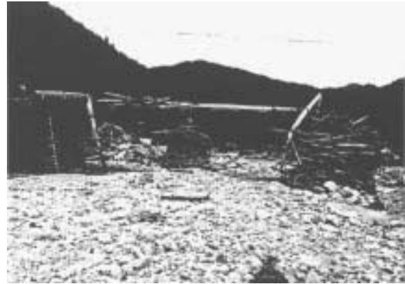
Photo. 1 Collapsed bridge washed away by the accumulated driftwood.
