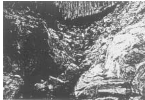
Photo. 4 Steep slope failure in Tappara, Kamiyahagi Town (lower part of the slope).
