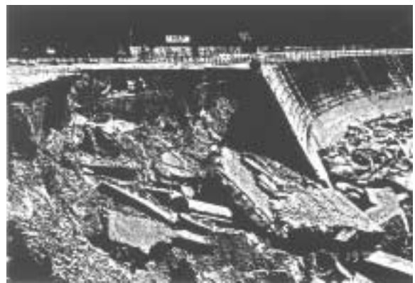
Photo. 2 Collapsed road and revetment washed due to scour of the retaining wall base.
