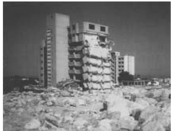
Photo 8. Building collapsed due to the direct strikes by boulders.
