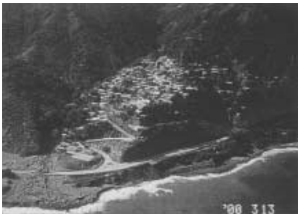
Photo 2. A shantytown on a very steep, weak slope.
