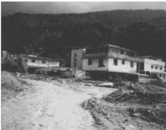
Photo 6. Destroyed houses at Carmen de Uria
