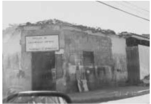
Photo 34. A confined masonry wall house in Santa Tecla.
