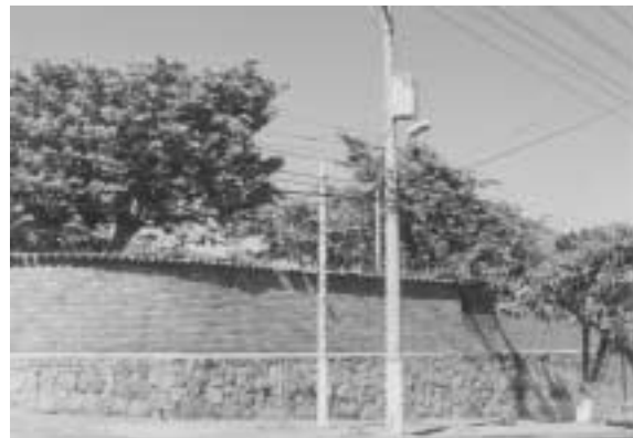
Photo 41. An un-reinforced masonry garden wall in San Salvador (no damage).
