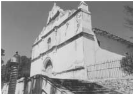
Photo 19. Damage to an adobe church in Zacatecoluca.
