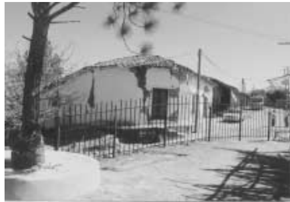
Photo 14. Damage to an adobe house in María Otsuma.
