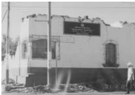
Photo 20. Damage to an adobe school in Usulután.
