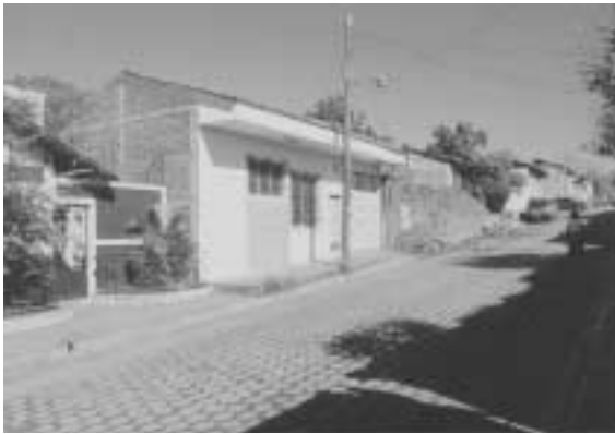
Photo 31. A confined masonry wall house in Usulután.
