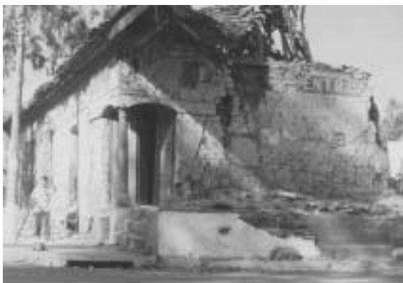
Photo 16. Damage to an adobe store in Santa Tecla.
