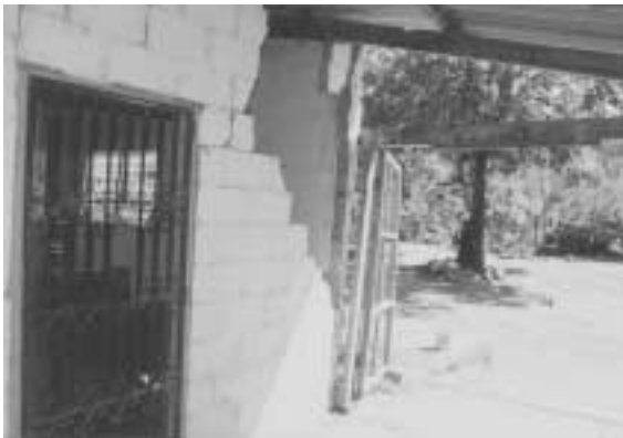
Photo 37. Failure of a hollow concrete-block masonry wall in the house in Photo 36. The hollow concrete block units are separated from the R/C confining column.
