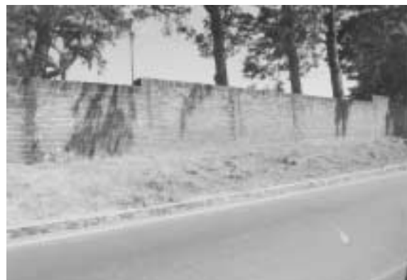
Photo 42. An un-reinforced masonry garden wall in San Salvador (no damage).
