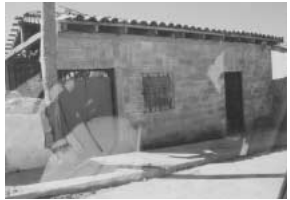
Photo 35. A confined masonry wall house in San Pedro Nonualco.
