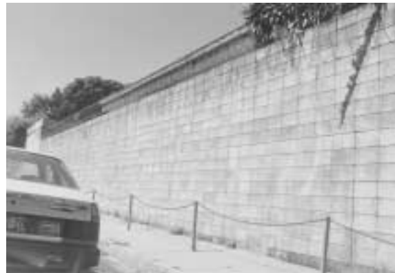
Photo 45. A reinforced masonry garden wall in Santa Tecla (no damage).
