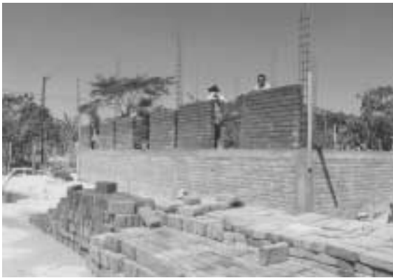
Photo 3. A confined masonry wall house under construction in La Paz Province.
