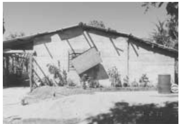
Photo 36. Damage to a confined masonry wall house in San Pedro Nonualco.
