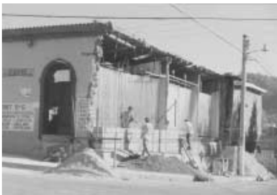
Photo 17. Damage to another adobe store in Santa Tecla.
