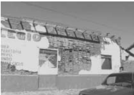
Photo 24. Damage to a mixed timber, bamboo, and mud wall school in Usulután.
