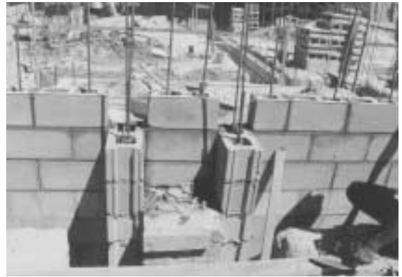
Photo 7. Reinforcing details of a masonry wall in the building in Photo 6.
