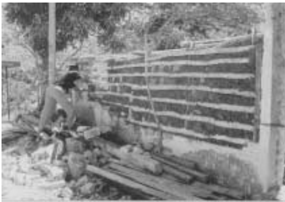
Photo 2. Mud filling work in the house in Photo 1.
