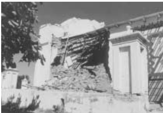
Photo 18. Damage to an adobe church in María Otsuma.
