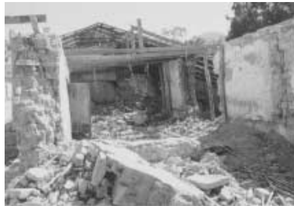
Photo 13. Failure of an adobe house in San Pedro Nonualco.
