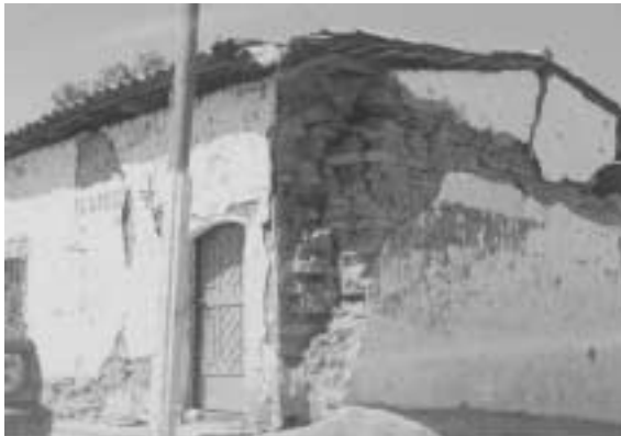
Photo 11. Damage to an adobe house in Santiago Nonualco.
