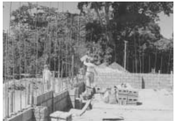
Photo 6. A reinforced masonry wall supermarket under construction in Santa Ana Province.
