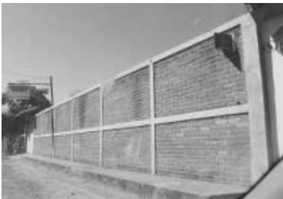
Photo 44. A confined masonry garden wall in Usulután (no damage).
