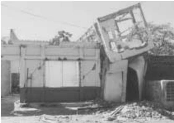
Photo 38. Damage to a confined clay-brick masonry wall in Usulután.
