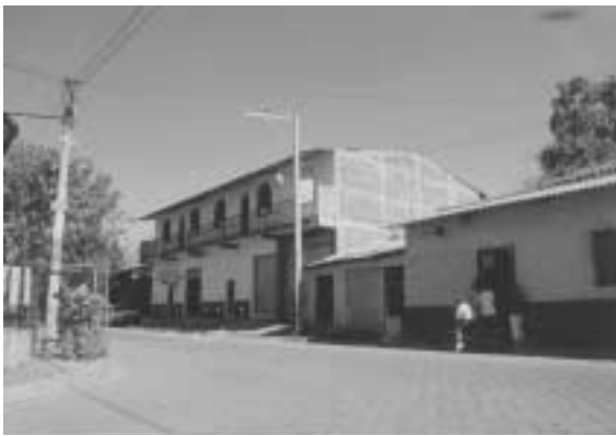
Photo 32. A two-story confined masonry wall house in Usulután.
