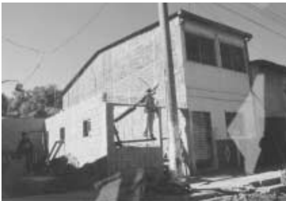
Photo 33. A two-story confined masonry wall house in Santa Tecla.
