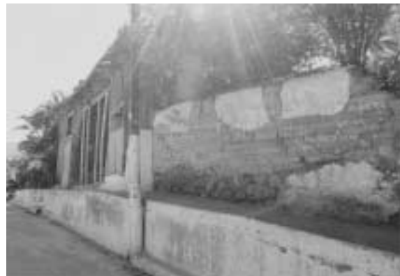
Photo 40. Failure of an adobe garden wall in San Pedro Nonualco.
