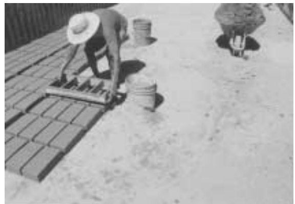
Photo 28. Forming clay bricks at the factory in Photo 27.
