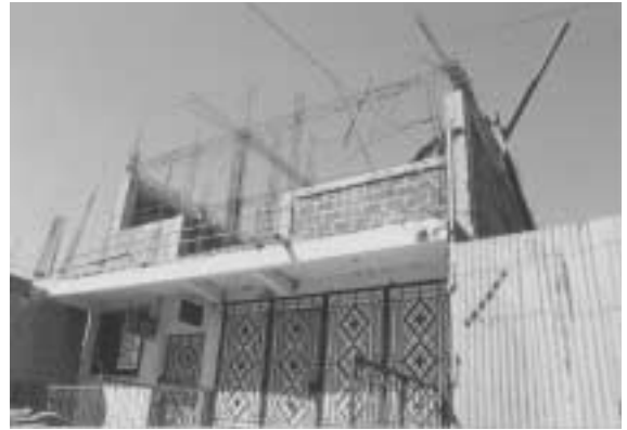
Photo 5. A confined masonry wall house under construction in Usulután.
