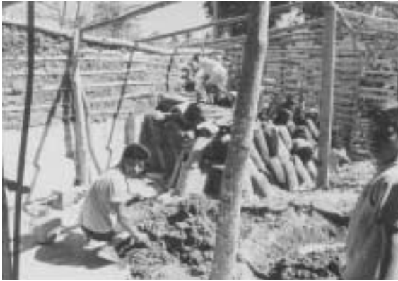
Photo 1. A mixed timber, bamboo, and mud house under construction in La Paz Province.
