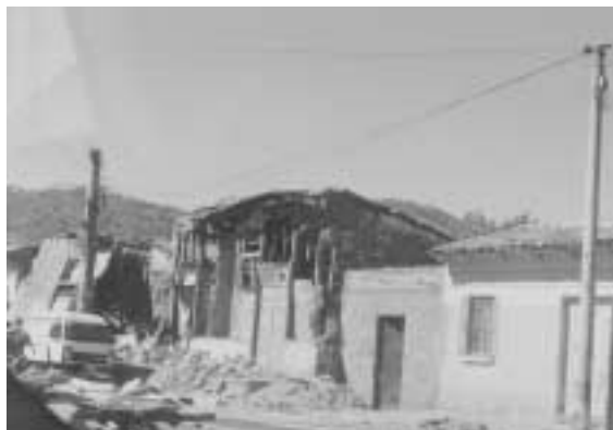
Photo 22. Damage to a mixed timber, bamboo, and mud wall house in Santa Tecla.
