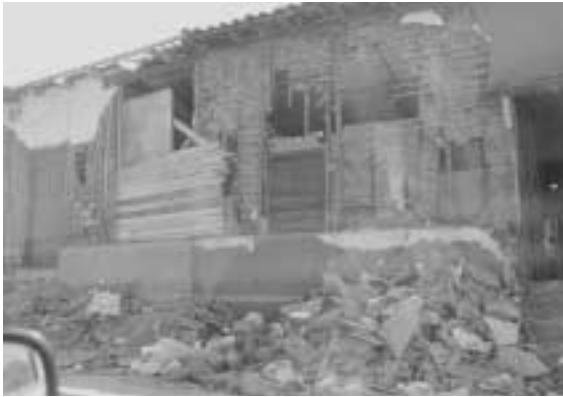
Photo 23. Damage to another mixed timber, bamboo, and mud wall house in Santa Tecla.
