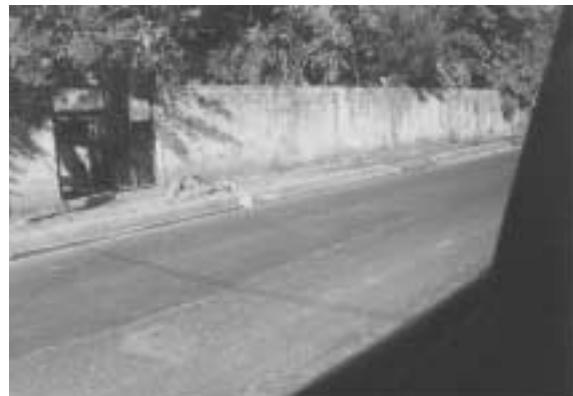
Photo 46. A reinforced masonry garden wall in Santa Tecla (no damage).
