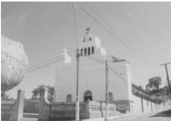
Photo 25. Damage to an un-reinforced masonry wall church in San Pedro Nonualco.
