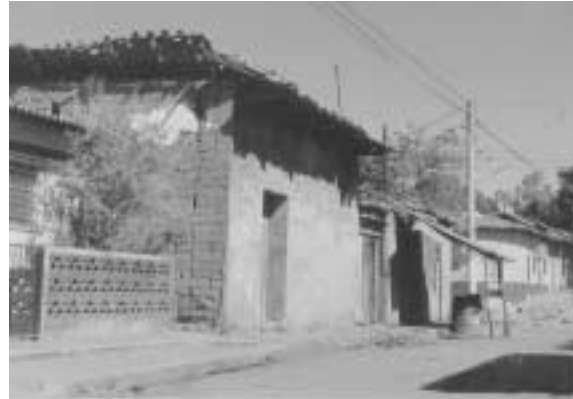
Photo 12. Vertical crack at the corner of an adobe wall in Usulután.
