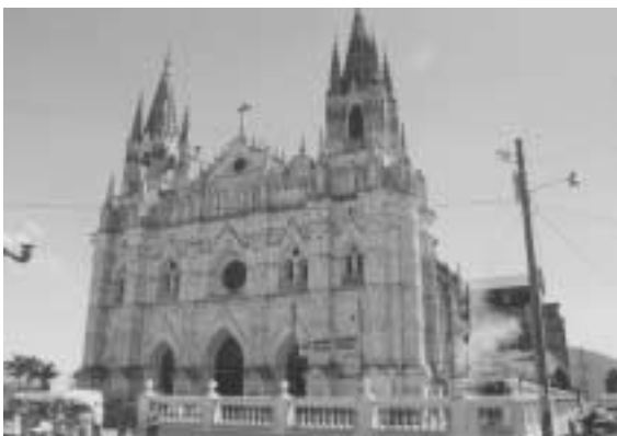
Photo 26. Slight damage to an un-reinforced masonry wall church in Santa Ana.
