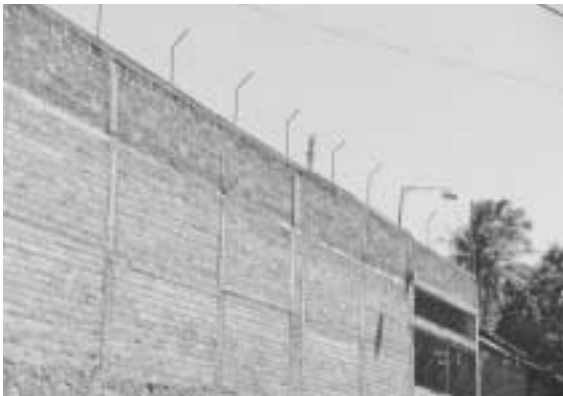
Photo 43. A confined masonry garden wall in Zacatecoluca (no damage).
