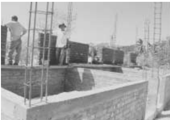
Photo 4. Reinforcing details of a confining column in the building in Photo 3.
