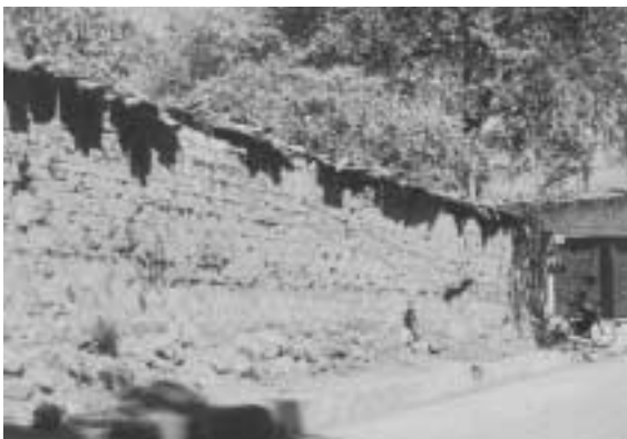
Photo 39. Damage to an adobe garden wall in Usulután.
