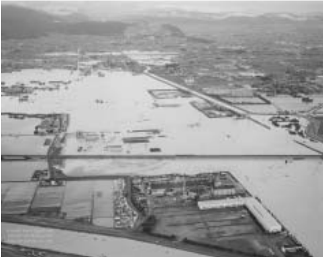
Photo 1 Flood damage in Ogaki City, Gifu Prefecture. Photograph: July 10, 16:00. The fuse plug levee is on the right. Copyright (C) 2002 Asia Air Survey Co., Ltd.
