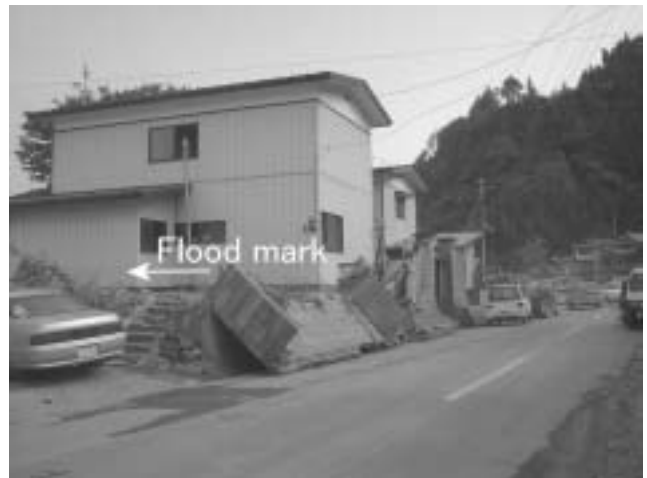
Photo 4 Inundated house in Higashiyama Town. Inundation by over flow in spite of being built on filled ground (about 1m). The wall was destroyed the river water. Photos 4, 5, and 6 were taken on July 13 by the author.
