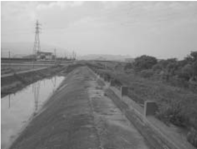
Photo 2 Close-up of the fuse plug levee (Otani River Arai zeki).
