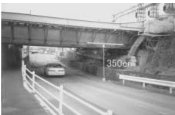
Photo 3. Flood mark under a bridge of the JR Tokaido Line (Yowa, Nishibiwajima Town).
