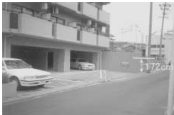
Photo 4. Flood mark on the wall of an apartment building located south of the JR Biwajima Station (Asahi-machi, Nishibiwajima Town).
