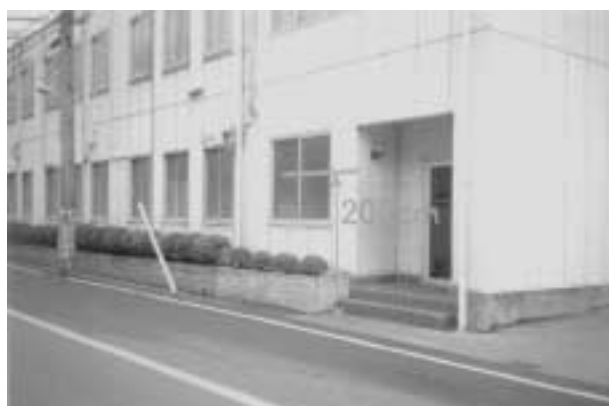
Photo 5. Flood mark on the wall of the building of Takaoka Electric Factory located about 500m west of Futatsuri Station on the Nagoya Railroad Nagoya line (Yoshino-cho, Nishibiwajima Town).
