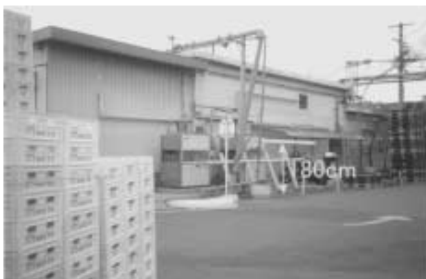
Photo 2. Flood mark on the wall of the Meito dairy factory located northwest of the JR Biwajima Station (Kaechi, Nishibiwajima Town).
