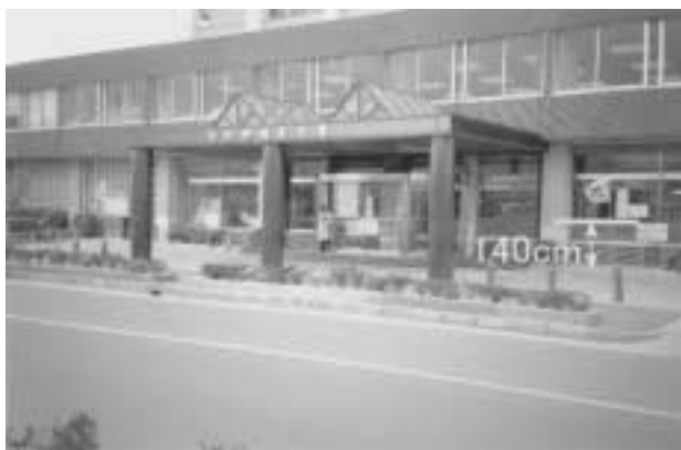
Photo 1. Flood mark on the glass of the door at the Nishibiwajima Town Office (Hanasaki-cho, Nishibiwajima Town).
